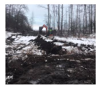
New culvert and drainage work on C4 near Hurricane and Cooper Roads. A minor trail re-location was completed here as well.
